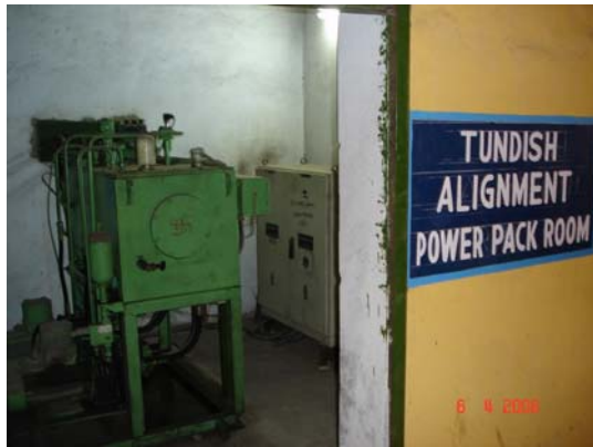
Fig 13: Hydraulic Power Pack and Main Electrical Panel
